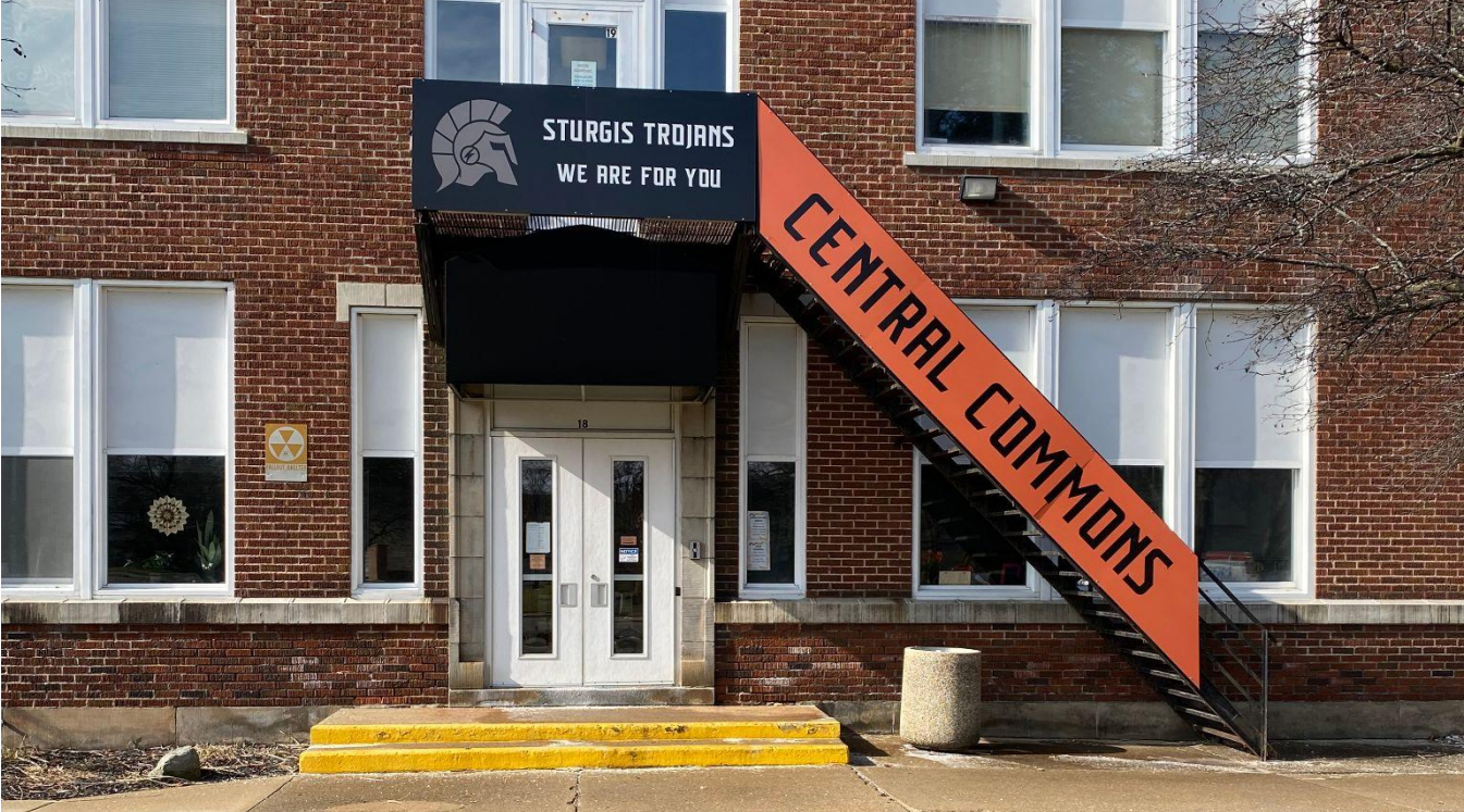
Pictured below: New signage on the fire escape at Central Commons.
