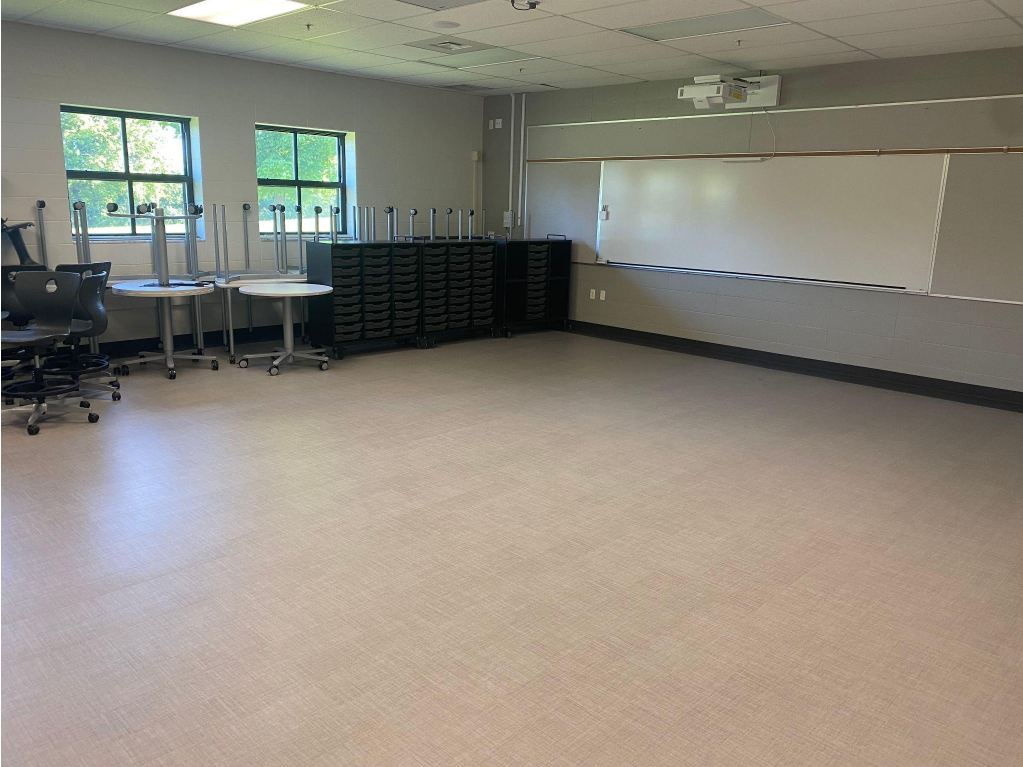
Pictured below: New classroom flooring.
