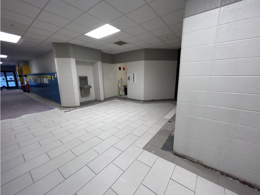
Pictured below: New hallway flooring being installed.
