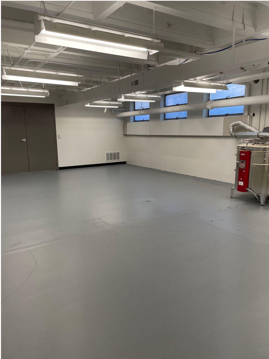
Pictured below: Lighting, HVAC, technology, fire code, and new wall complete.
