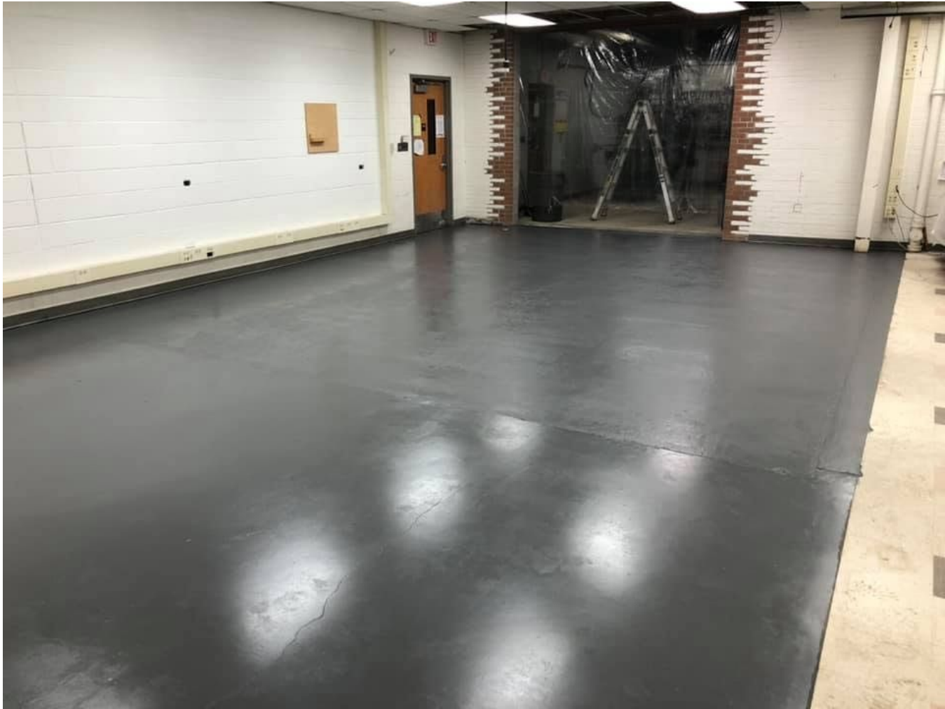
Pictured below: New flooring in expanded shop.
