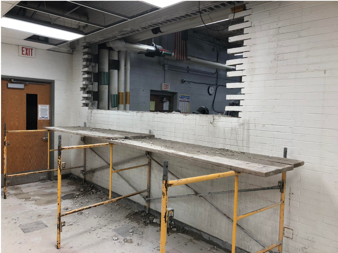
Picture below: Wall being removed.
