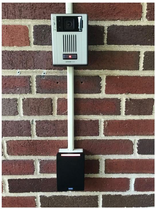
**Update 8/22/2019:** The new card readers and intercoms have by installed on an exterior wall alongside the old system as the new system is getting hooked up.
