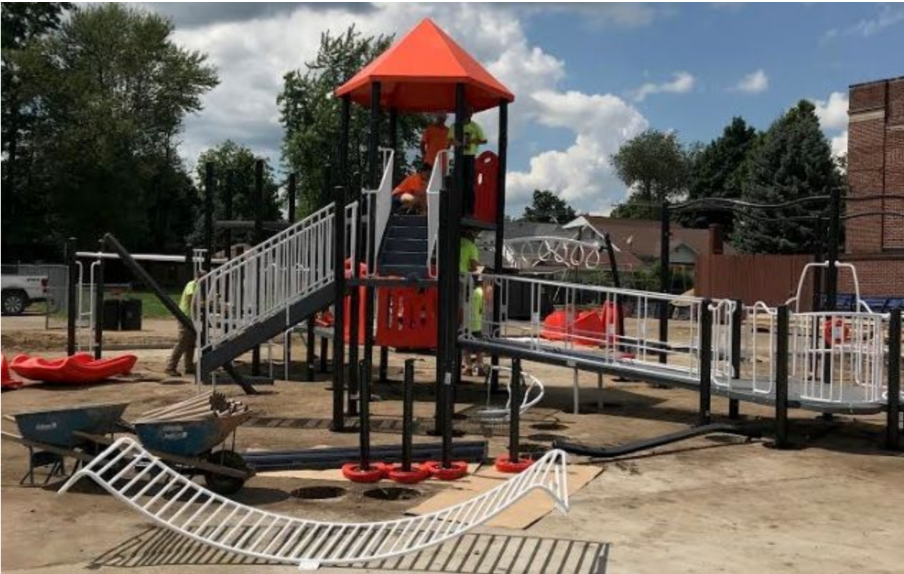
Update: 7/30/2019: Crews continued installation of the play structures.
