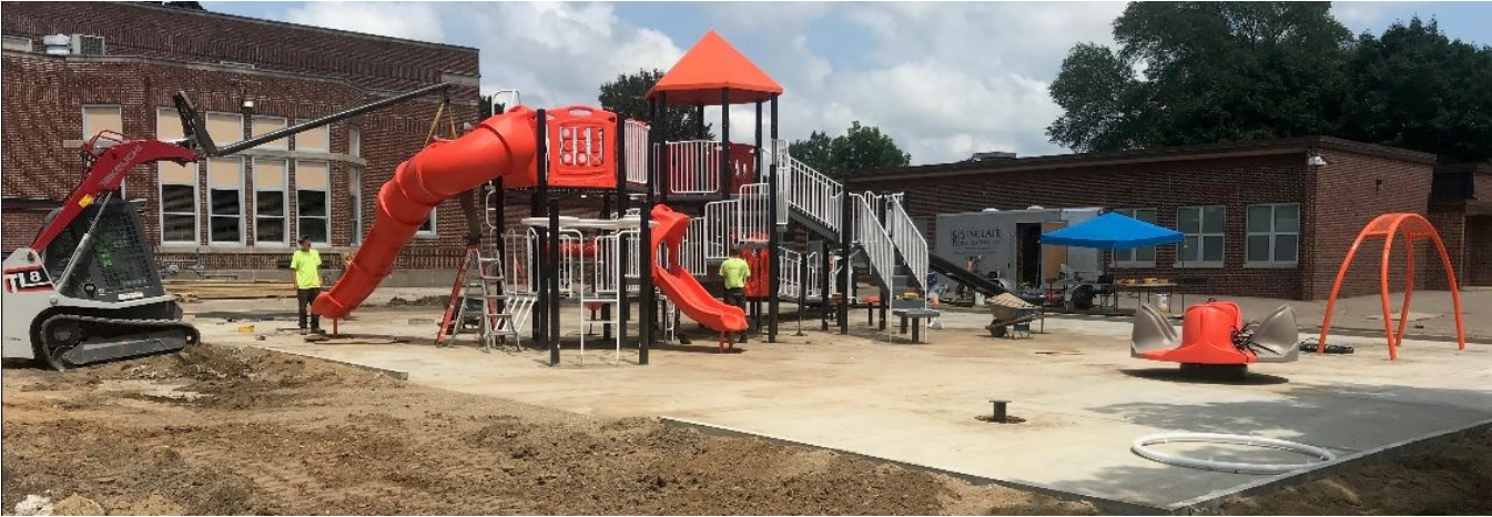
Update: 7/31/2019: Crews continued installation of the play structures.
